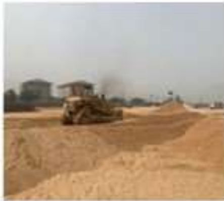
Sand-filling / Compaction - ongoing
