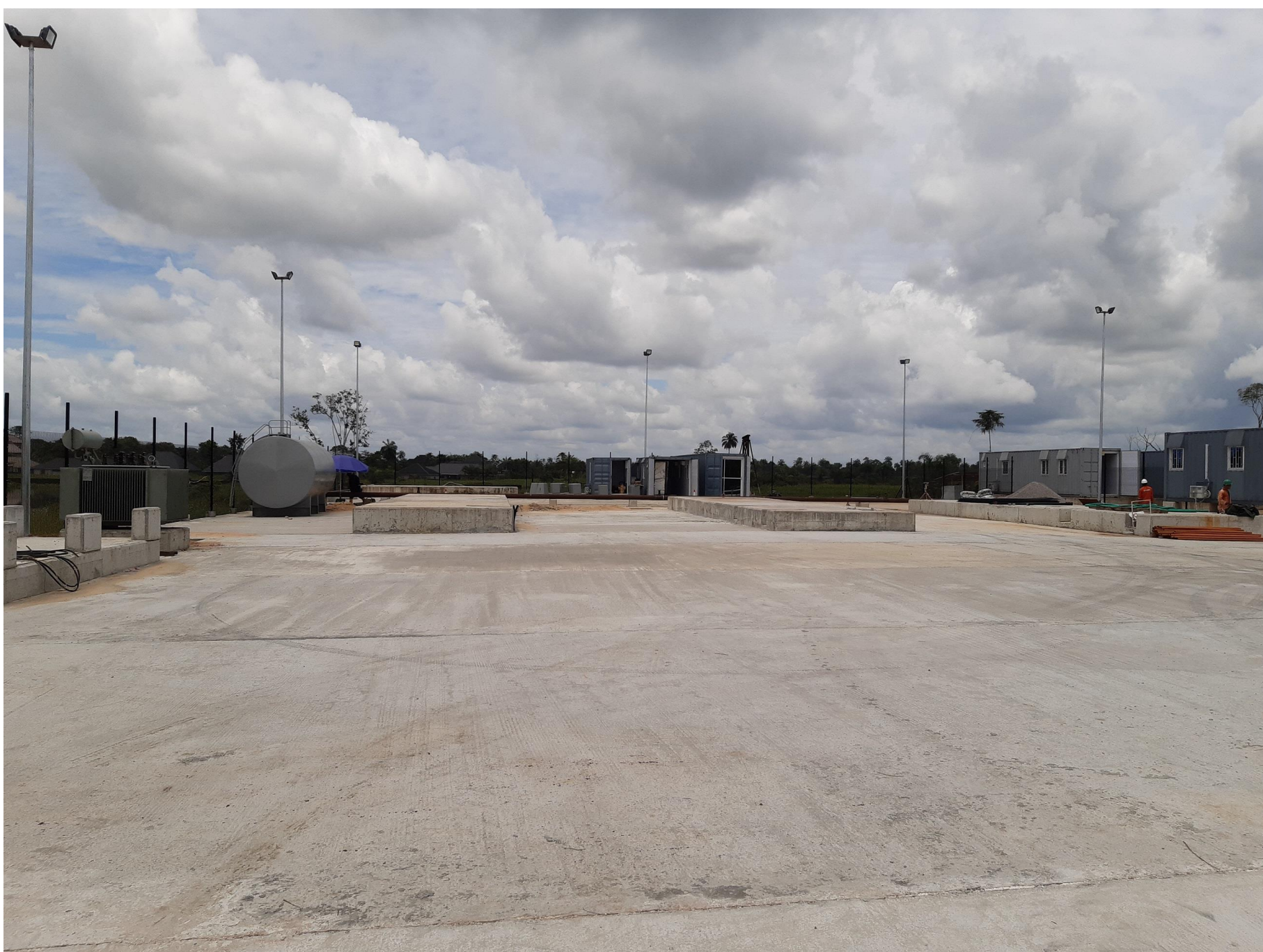
View of the Foundation Pads for the Gas Turbines
