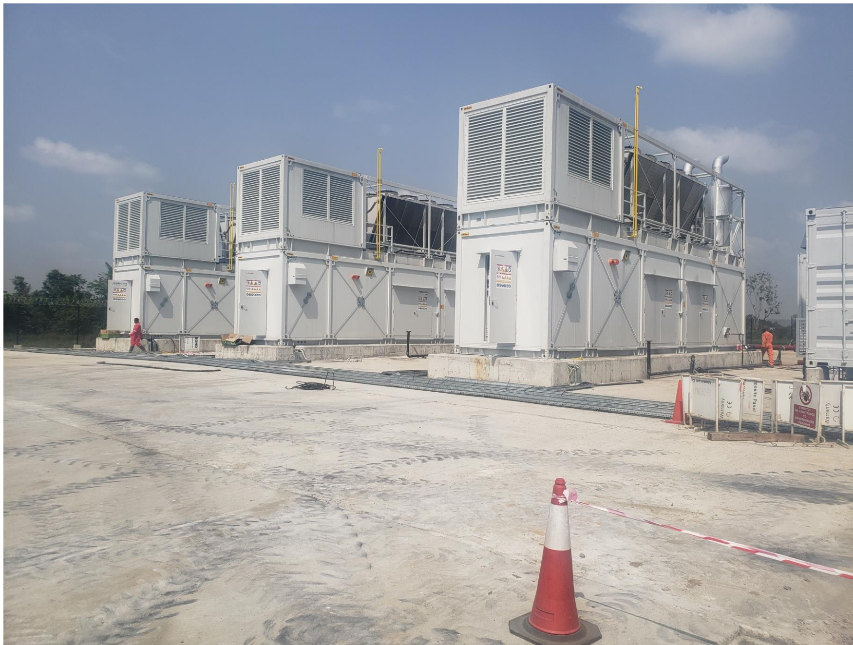
View of the Installed Gas Generators with Combined Capacity of more than 10MW
