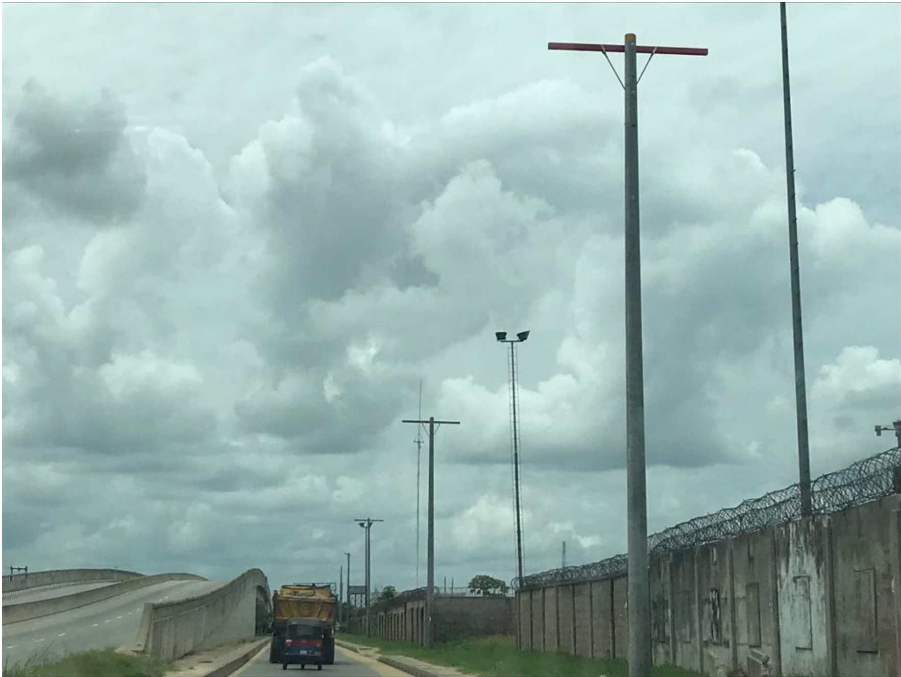
Installed Reinforced Concrete Electric Poles that will carry 33Kva Power Lines to HQBP Site
