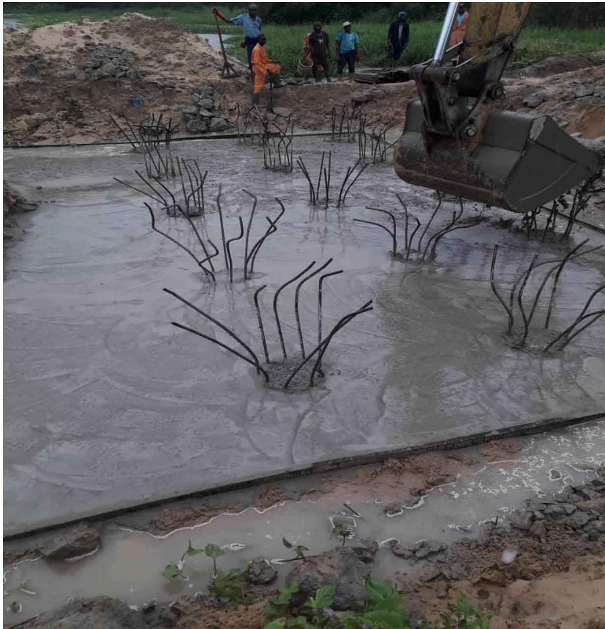
Foundation Work for Bored Cast in Place Piles
